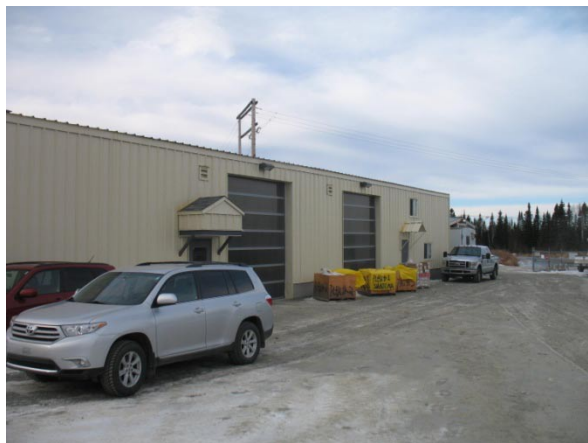
Building with core logging and cutting facility
