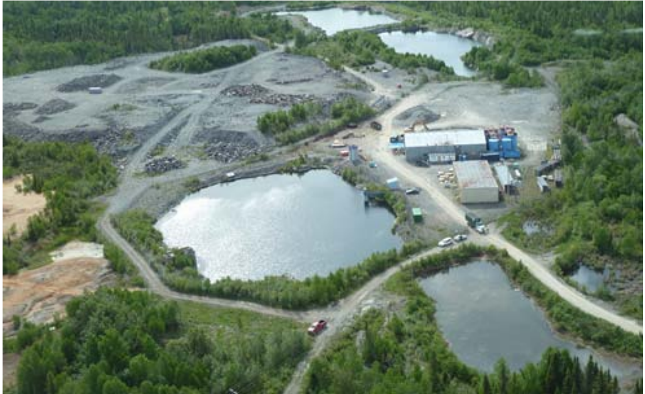
Figure 8: Air view of existing infrastructures looking South-East (in 2010).
