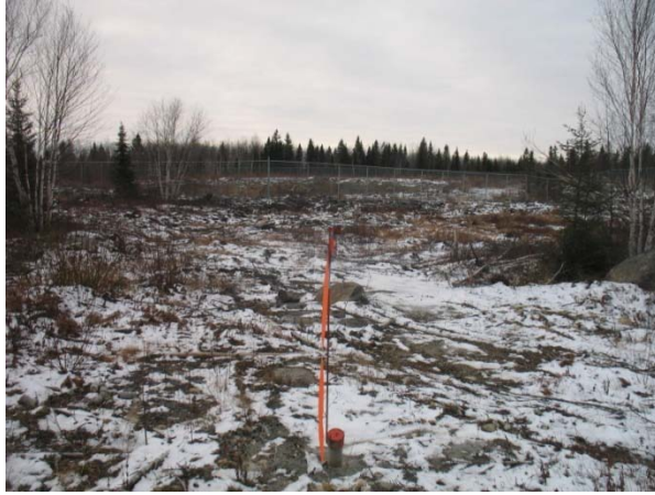
Drill site with identified casing 2011 pit fence in the back
