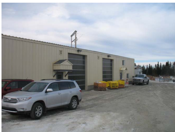
Building with core logging and cutting facility
