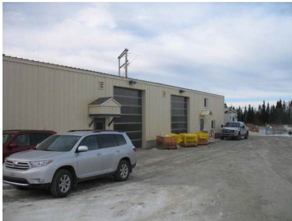
Building with core logging and cutting facility
