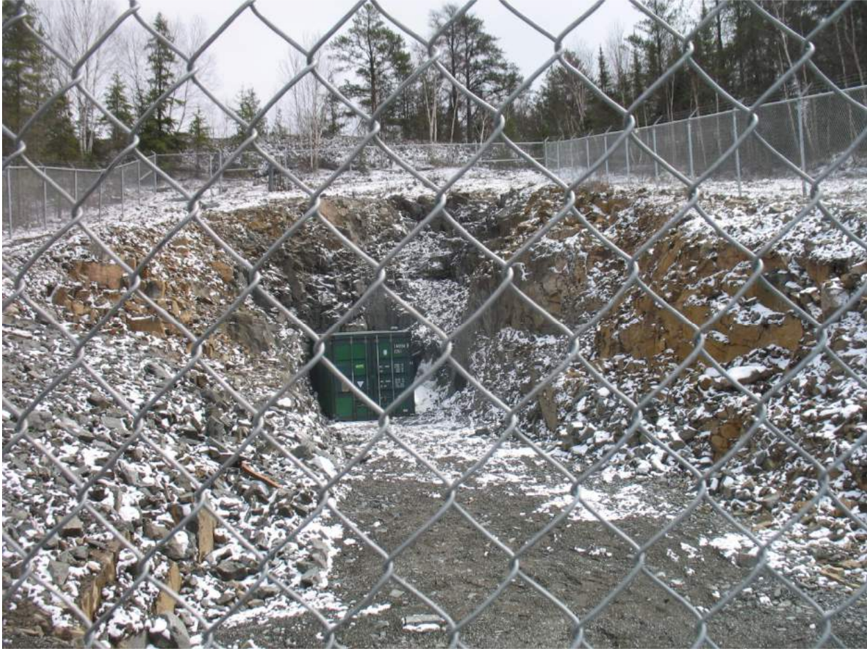
Figure 38 : Rehabilitation and protection of the adit entrance
