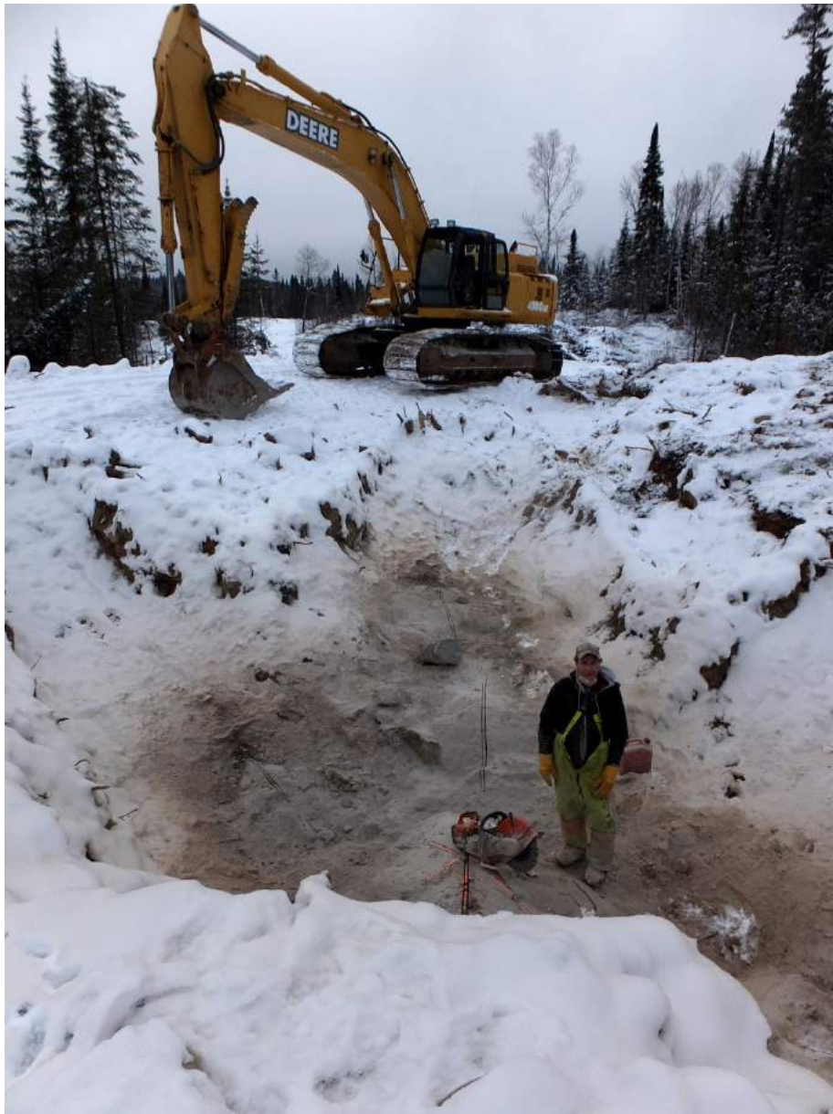
Figure 24: winter trenching program
