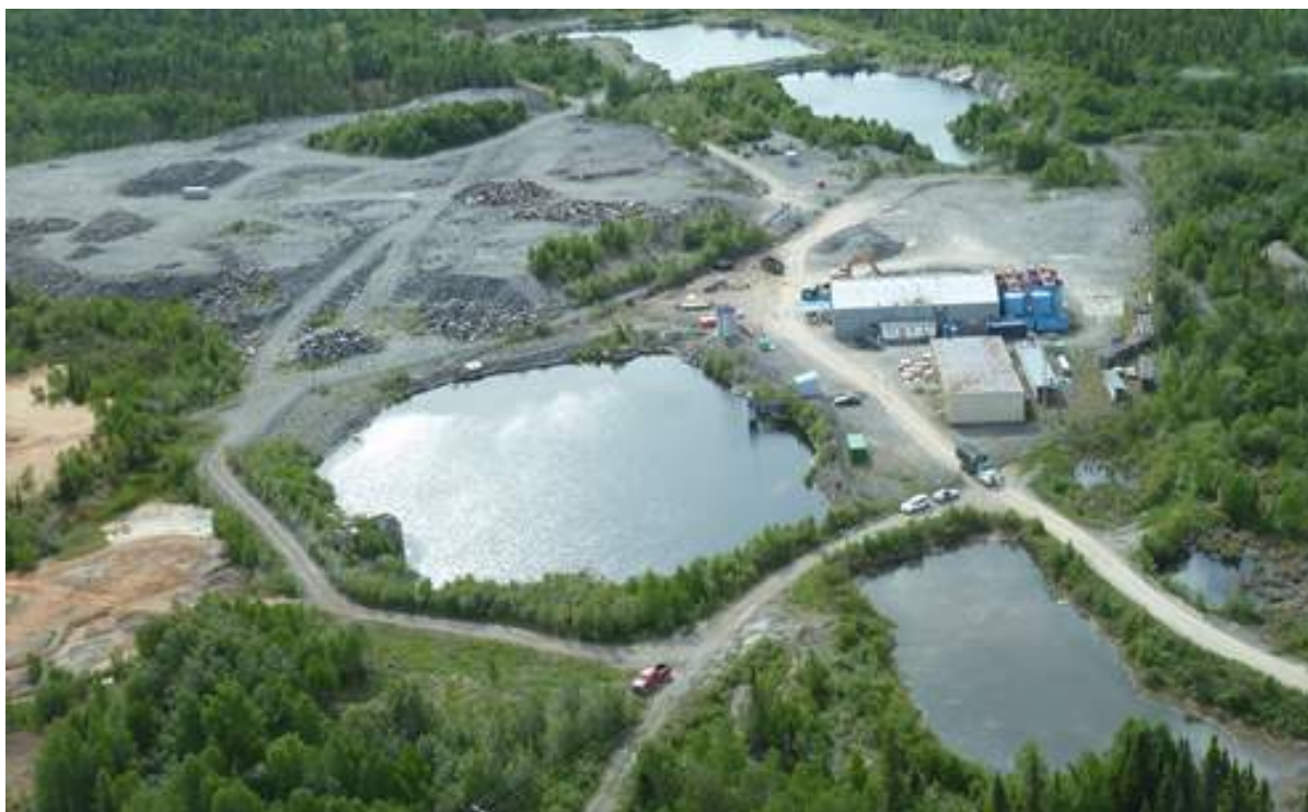
Figure 5: Air view of infrastructures looking South-East (in 2010)
