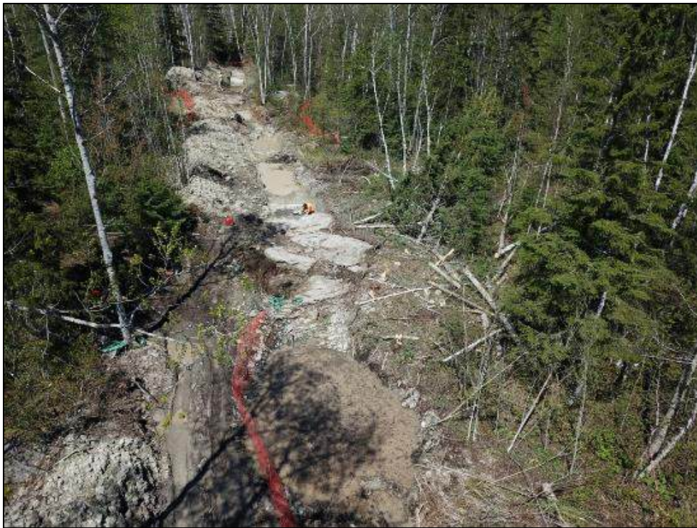
Figure 9-3 Trenches at Aukeko Site
