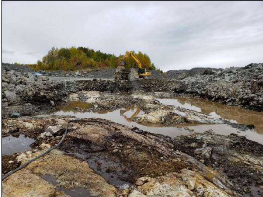
Figure 9-6 2019-2020 Stripping on Granada Property
