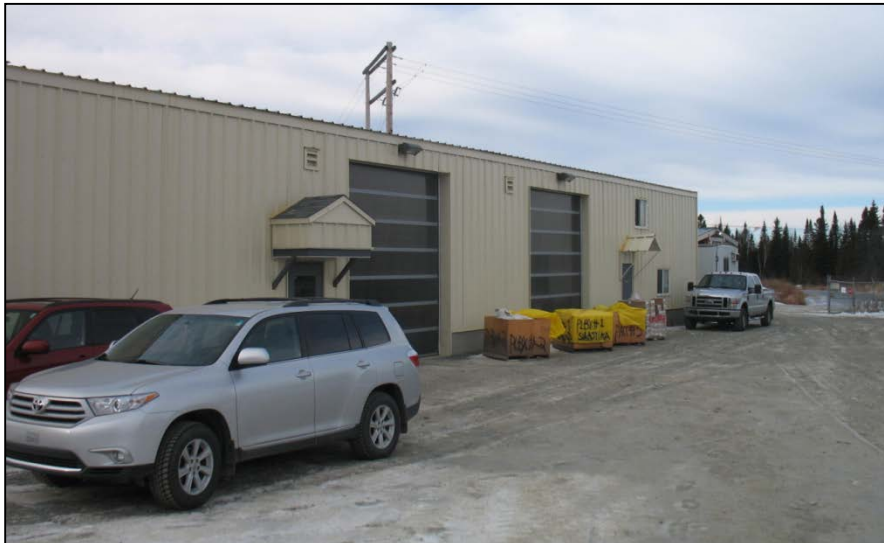
Figure 18-3: Existing on-site infrastructures
