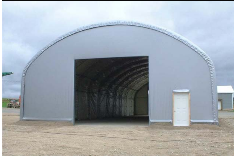
Figure 18-4: Example of a dome type mechanical garage
